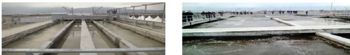
Figure 2. Appearance of the purification plant in city Strumica
