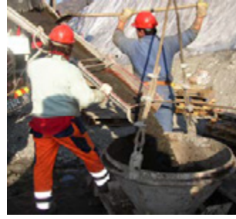
Fig. 2 ZVI poured into the excavation
