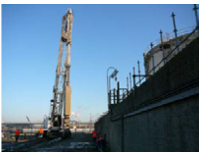
Fig. 5 Slurry wall excavation
