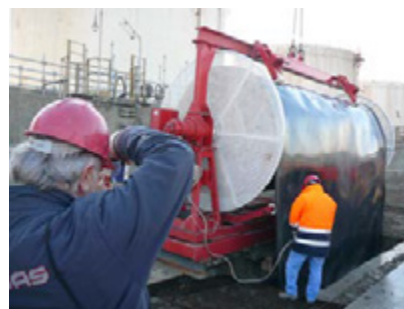
Fig. 6 HDPE liner placing drum
