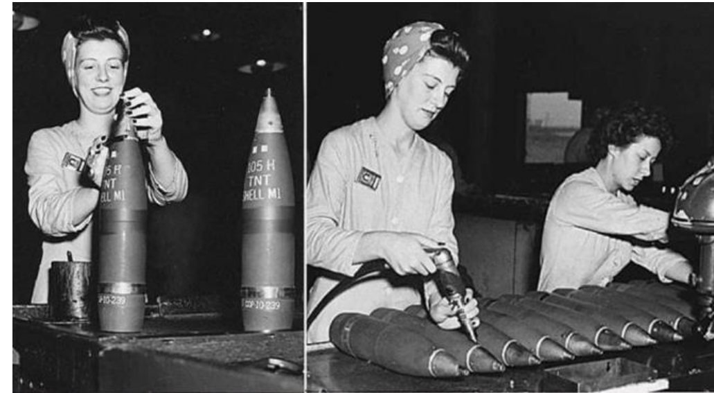
Beryllium tools were the norm in munitions industry. These were typically 2% copper Beryllium alloys, used for avoiding spark.
